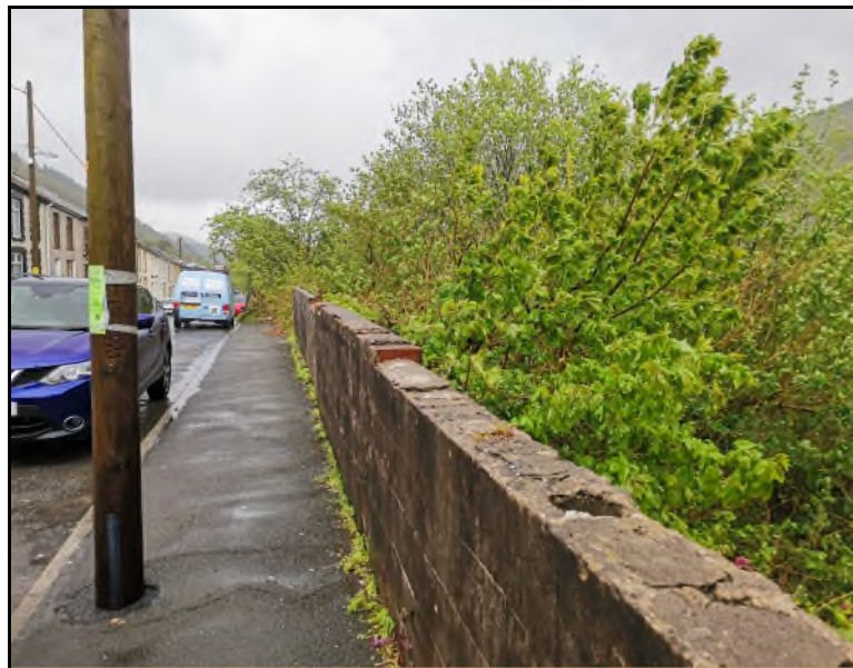
Fig. 3 - Application Site (looking southwards)
