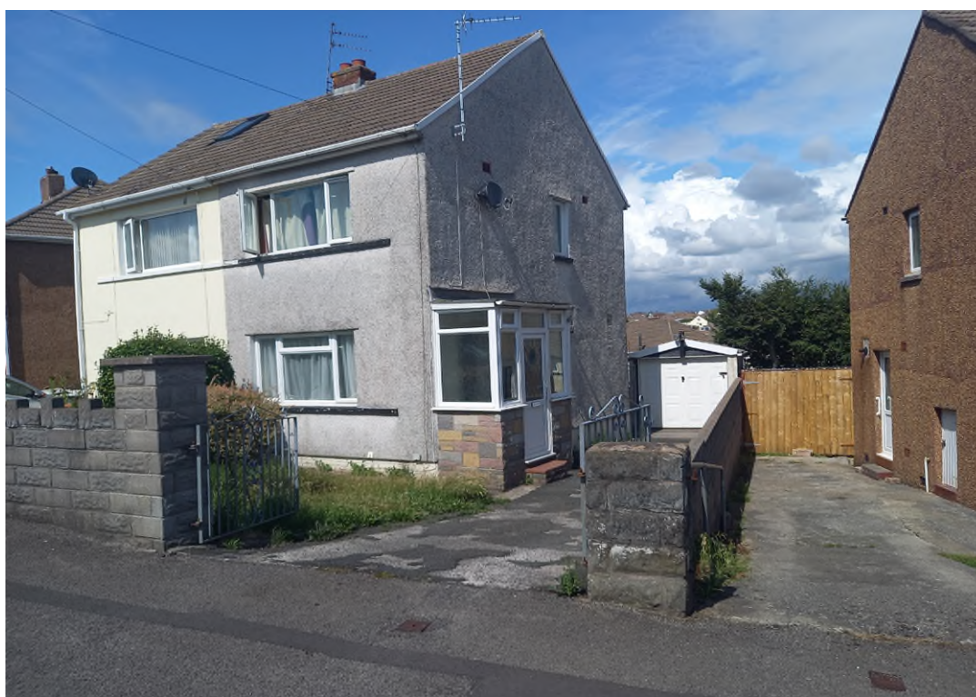
Figure 1 - Photograph of Existing Property:
